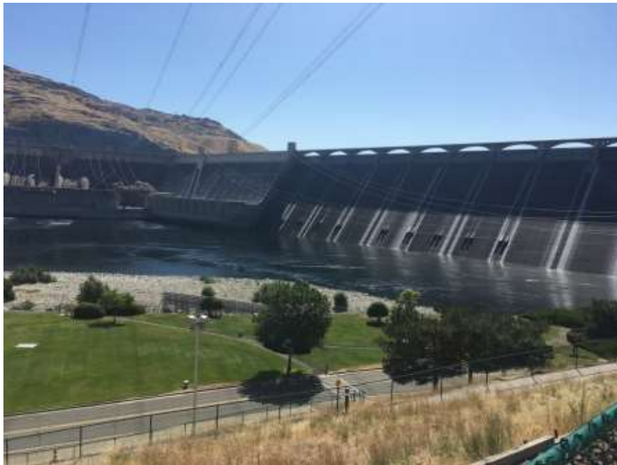
Grand Coulee Dam
