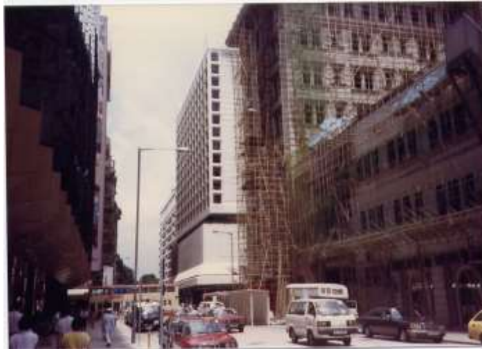
Bamboo scaffolding in Hong Kong
