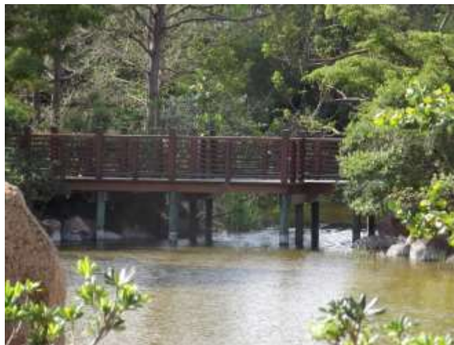
Twisted bridge from across lagoon
